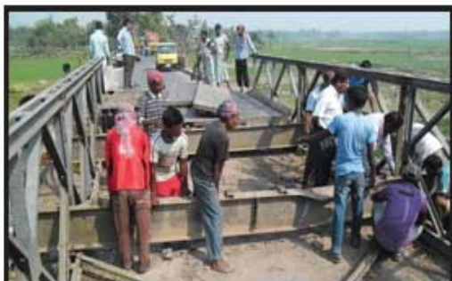
The workers are repairing the bridge.
